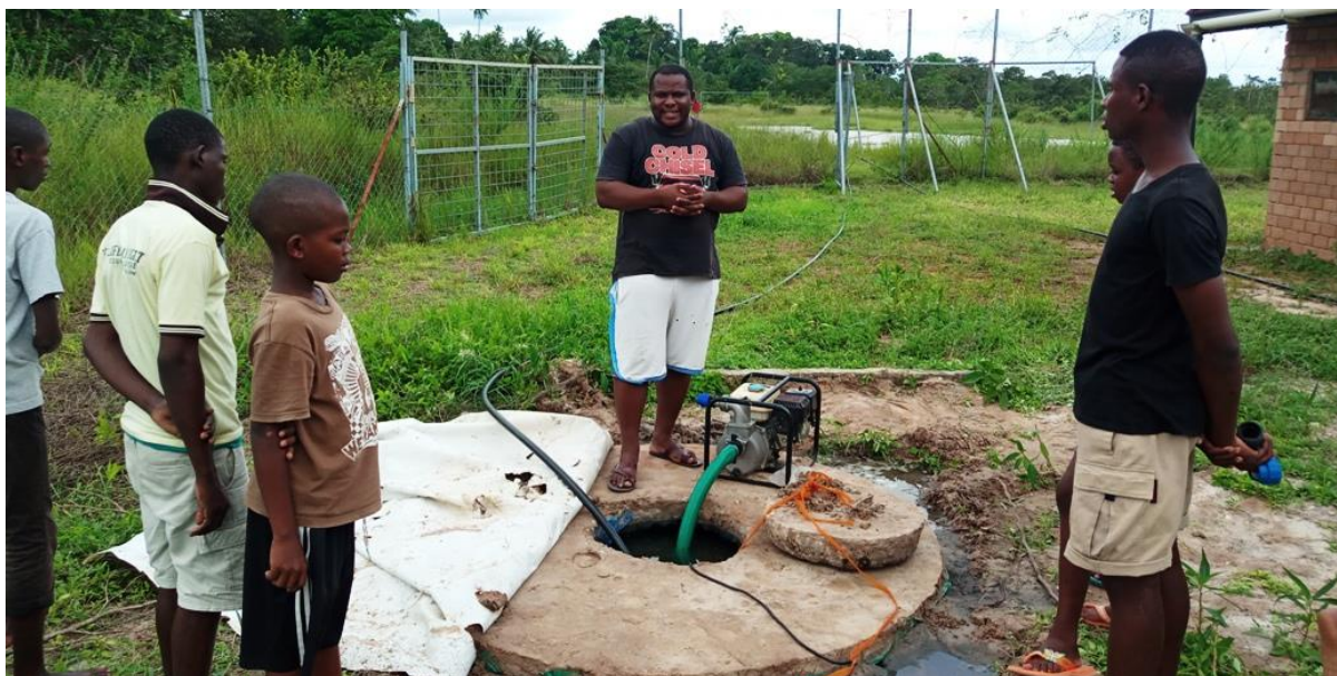
Fixing the water pump
